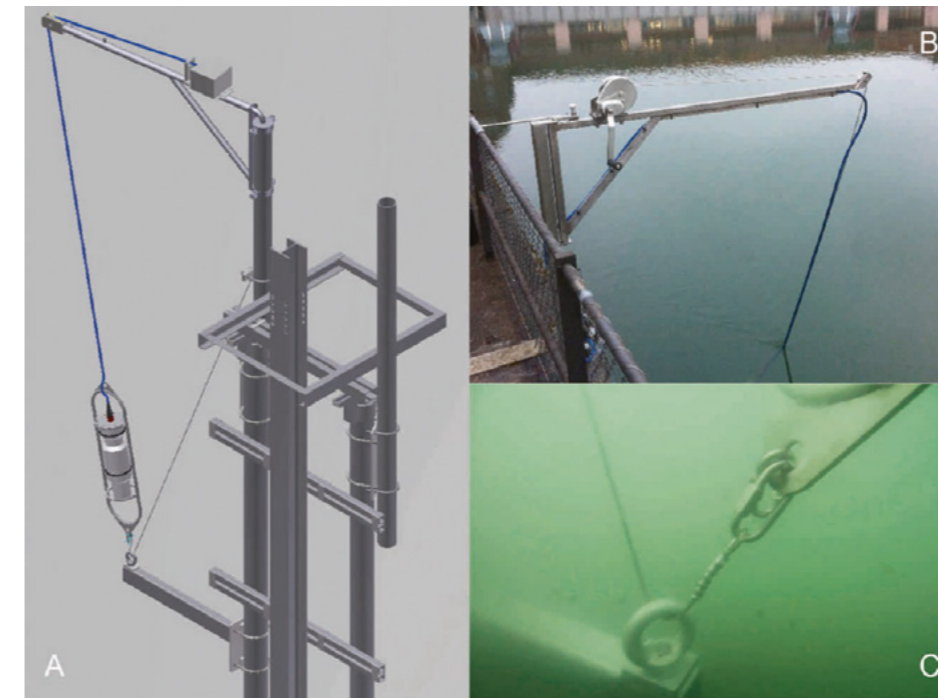
Figure 5 A) Plan for installing a water probe on an underwater structure; B) A hoist mounted on the riverbank; C) The lower anchoring system. The hoist holds the blue connector cable and the supporting steel cable in place underwater. The lower steel cable is used to position and secure the probe (Image A: D. Wyder, Metas; Image C: taf-taucharbeiten ag)
